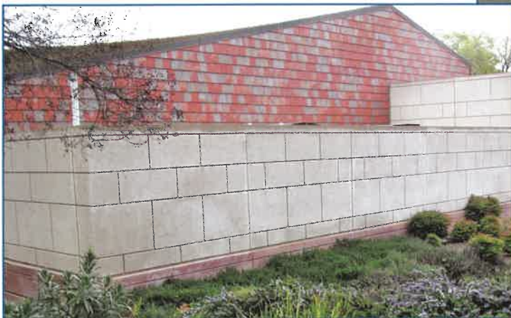
Figure 1 – Boiler room has perimeter cast-in-place concrete walls (commencing below the reddish precast panels) extending down to the concrete footings. (Whitish precast concrete panels extend up from the red panels.)
