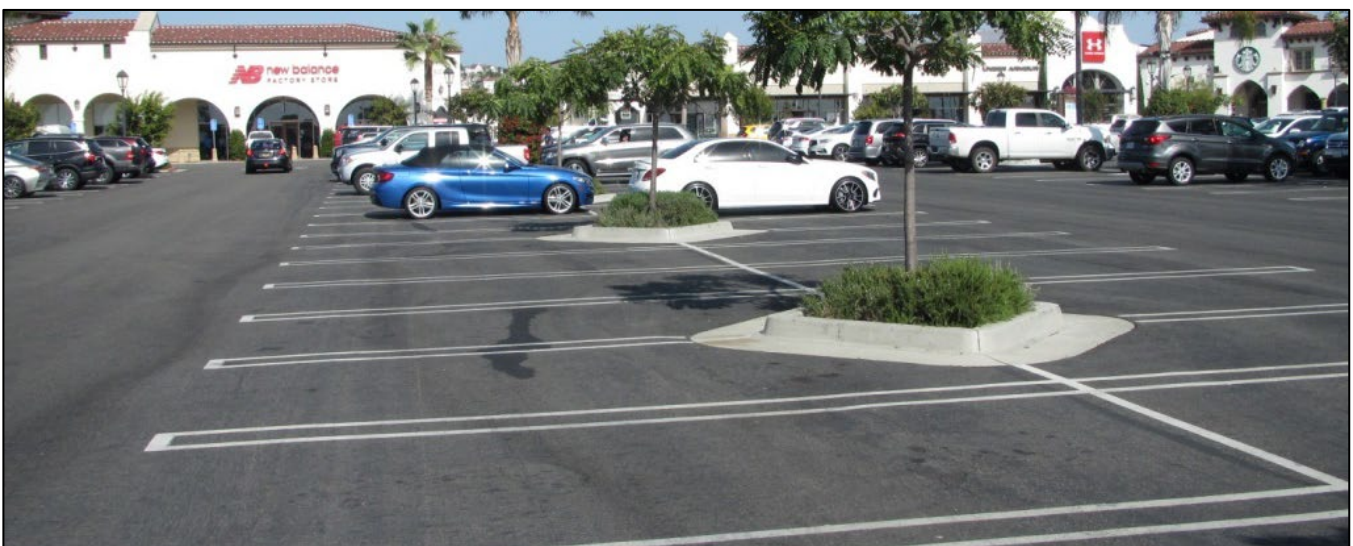
Photo 5 – Designers of this Southern California parking lot similarly elected to eliminate wheel stop tripping hazards.
